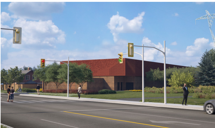
Traction power substation on McCowan Road in the Hydro corridor (view looking east)
