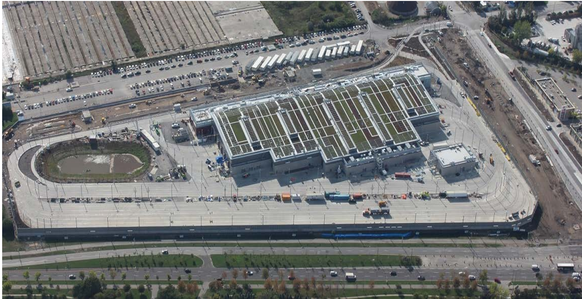
Aerial view of the Leslie Barns Streetcar Facility
